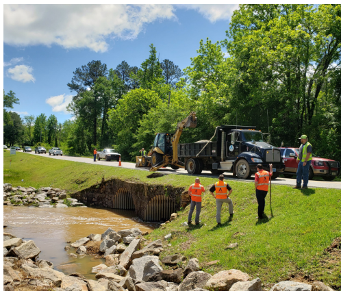
Crews work to repair a culvert after heavy rains in April.
